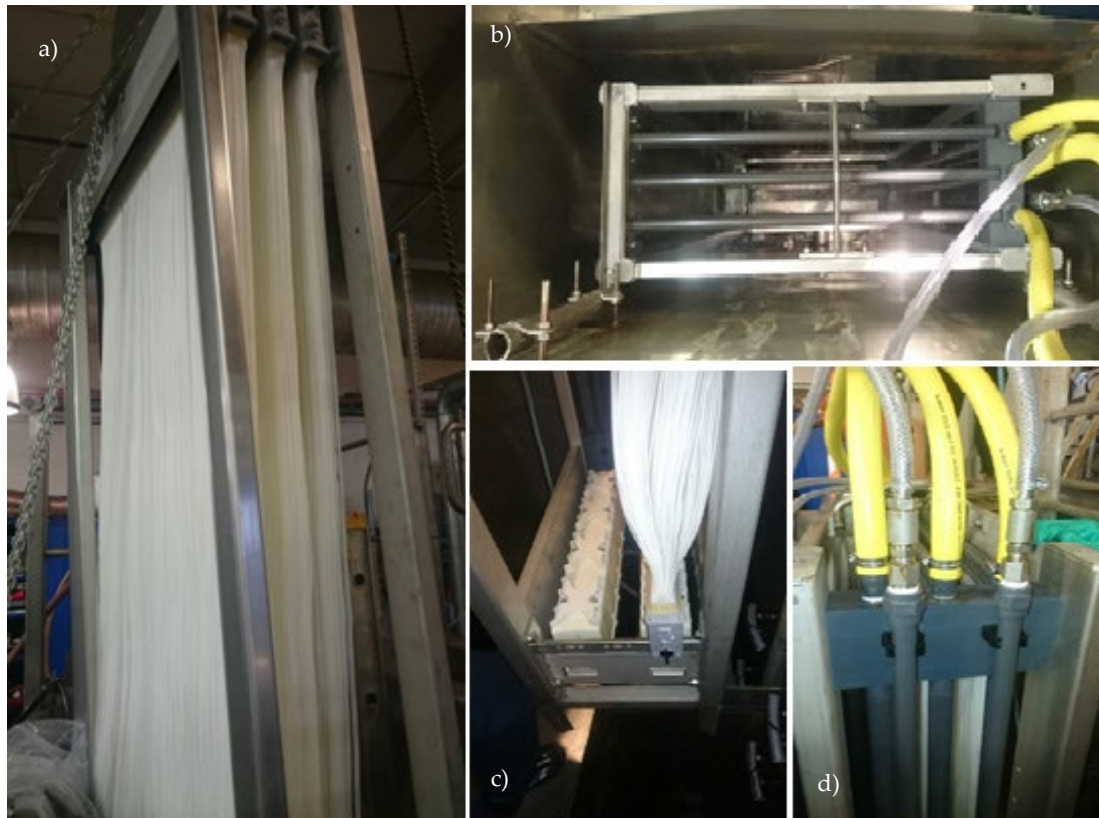
Figure 5. The membrane during installation of the pilot. a) Membrane cassette with three membrane modules, b) cassette lowered into the tank, view from above, c) mounting and aeration equipment at the bottom of the cassette, d) permeate connections (yellow) at the top of the cassette.
